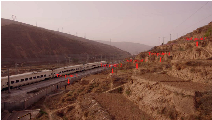
FIGURE 2: Field test overview.
