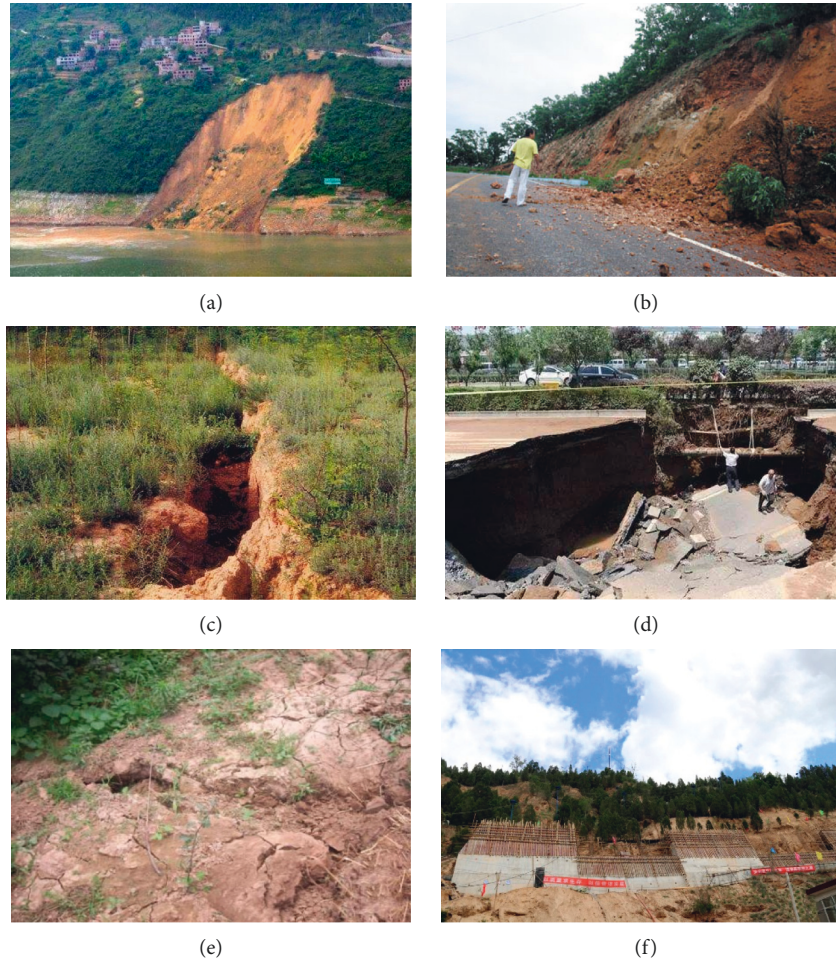
FIGURE 3: Common types of loess disasters: (a) loess landslides; (b) collapses; (c) loess collapsing; (d) ground collapse; (e) ground fissures; (f) unstable slopes.
