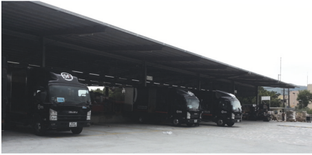
FIGURE 6: The docks and trucks at the DC.
