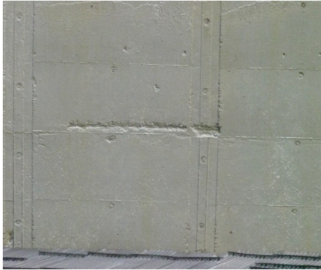
FIGURE 3: Concrete after maintenance.
