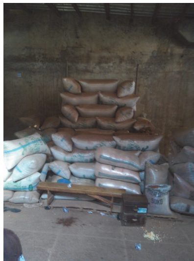
FIGURE 1: A typical foodstuff warehouse showing the roof without vents.
